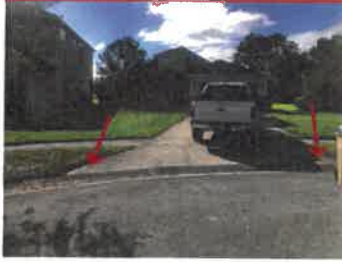
209 WESTMORELAND CIRCLE Decorative markings on driveway
