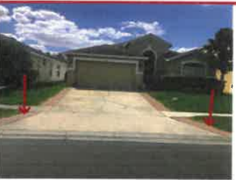
945 TRAMELLS TRAIL Paver expansion
