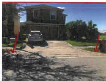
245 OWENSHIRE CIRCLE Pavers added both sides of driveway
