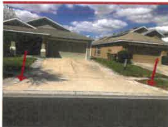
2711 LUCAS LAKES Driveway expansion pavers
