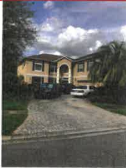
232 STRATHMORE Pavers installed
