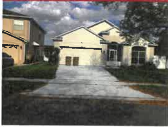
131 HARWOOD CIRCLE Paint/stain
