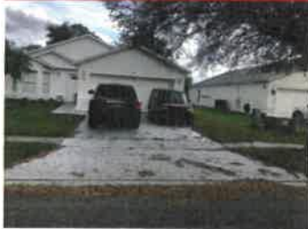
184 HARWOOD CIRCLE Paint/stain
