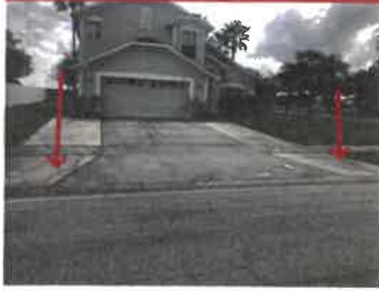
162 BURRELL CIRCLE Concrete added to sides of driveway
