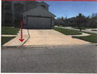
201 STONE CROFT CT Driveway modification
