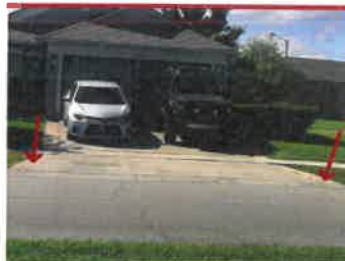
2400 KNIGHTSBRIDGE Pavers on side of driveway
