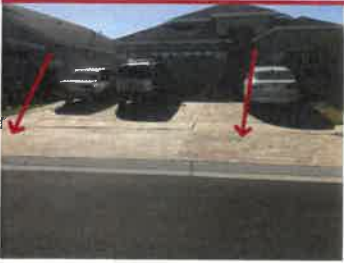
969 TRAMELLS TRAIL Paver extension both sides of driveway
