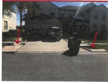
107 SOUTHAMPTON Modifying Driveway on each side
