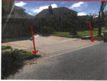
192 WESTMORELAND Pavers on side of driveway
