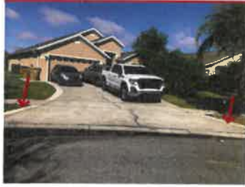
155 SOUTHAMPTON Driveway modification concrete
