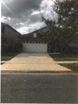
118 HARWOOD CIRCLE Decorative markings
