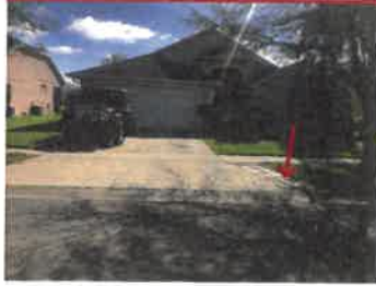
113 SOUTHAMPTON Pavers on side of driveway
